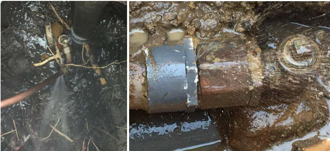
Figure 2 (left): Service line leak at the connection to the main. Figure 3 (right): Leak on PVC main
