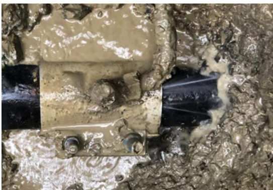
Figure 37: five days after leak was repaired the main was dug up revealing the failed repair.
