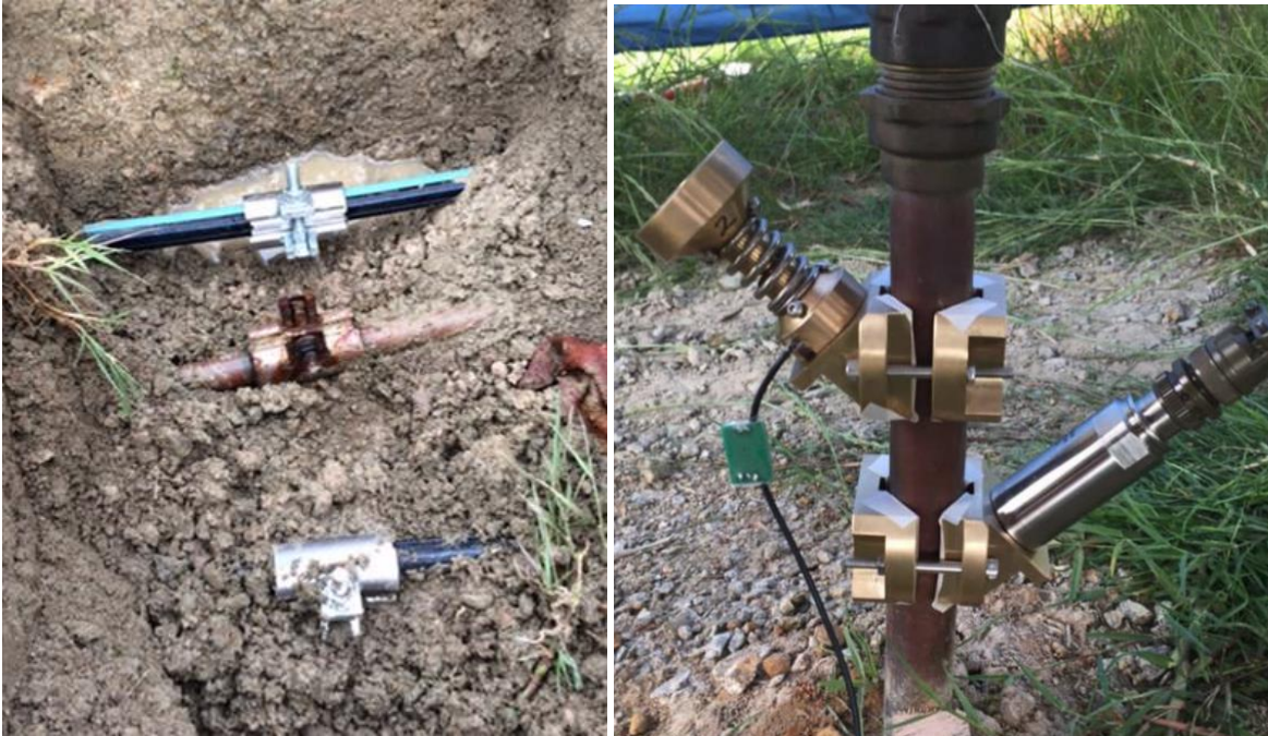
Figure 7 (left): exposed pipes where leaks were created by drilling. Figure 8 (right): prototype sensor and Meggitt Mems sensor used as a reference mounted to the test pipe
