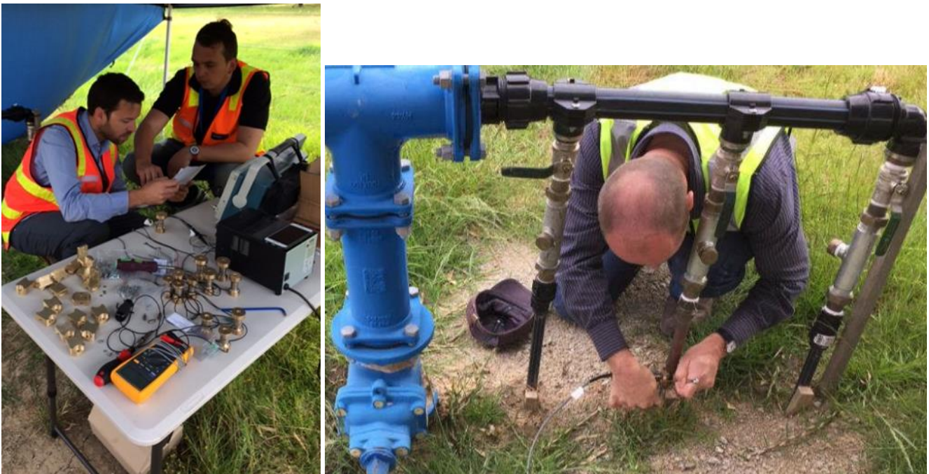
Figure 5 (left): test rig instruments and prototypes. Figure 6 (right): installing mount pipe for prototypes
