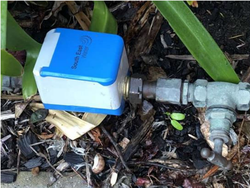
Figure 24: Digital water meter containing the vibration sensor deployed on a residential property.
